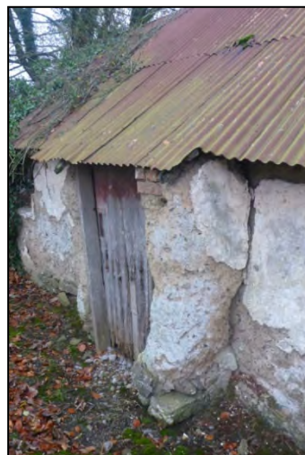
Plate 15-10 Vernacular structure BH4, close-up of porch
