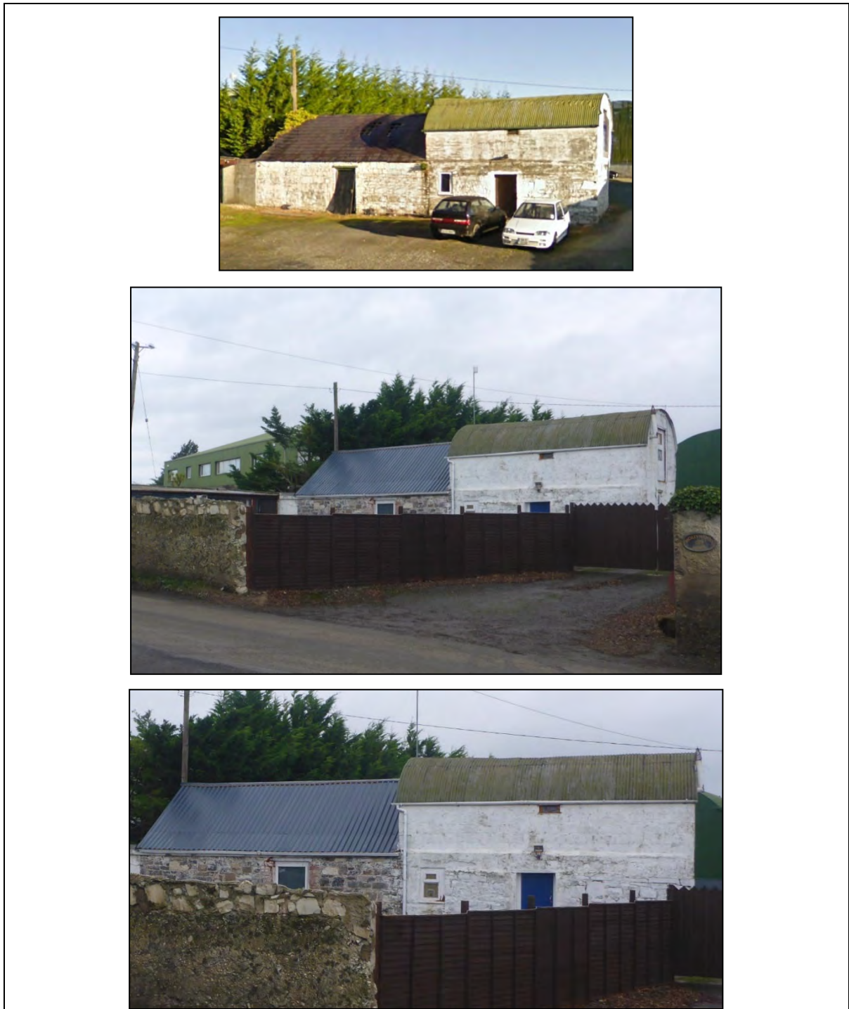
Plate 15-7 Farmstead BH2: Vernacular structures on site visit (above and middle) and in 2010 (top; Google image)
